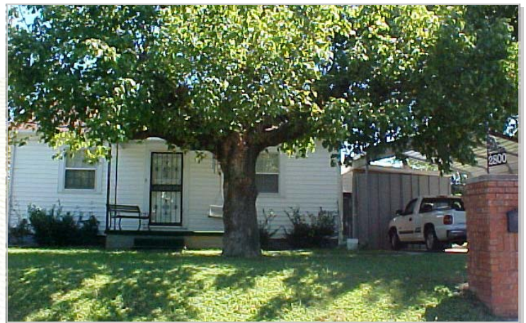
S. Hawthorn Street Single-Family Residence
