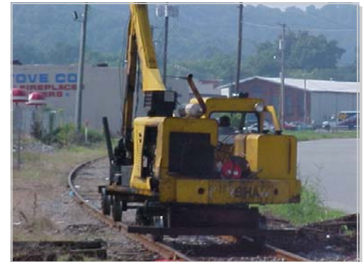
Railroad maintenance between Rossville Boulevard and State Street.
