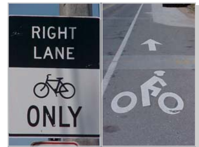
Bike lane signage and pavement marking as seen on Clio Avenue.
