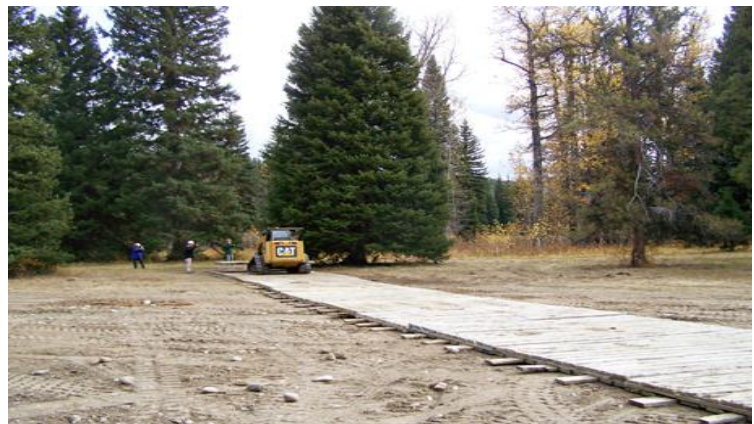
Figure 5.2.1-10. Using wood mats to protect soil from compaction.
