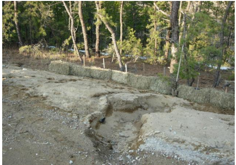
Figure 5.2.1-8. Soil protection at woodland edge.
