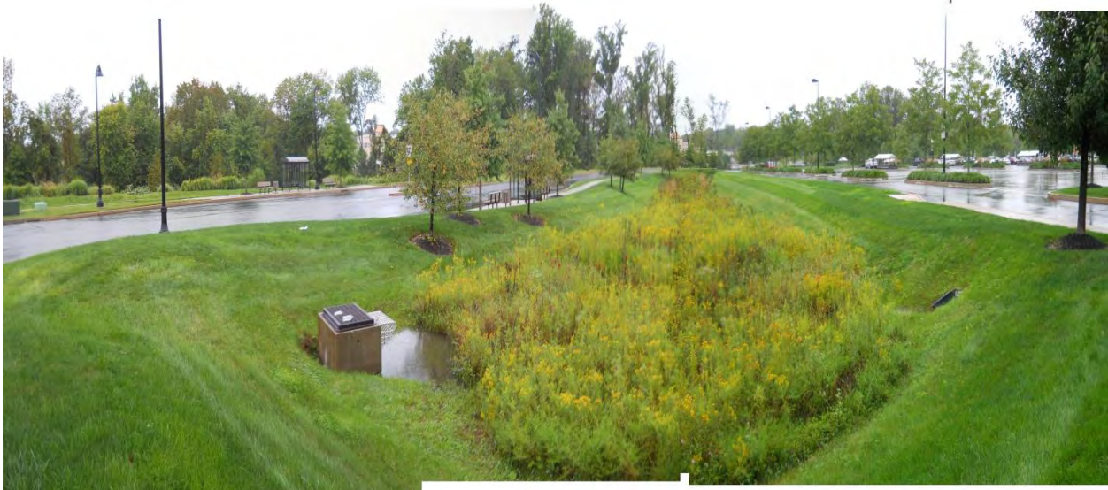
Figure 5.3.13 -4. This naturalized basin captures runoff from a high traffic roadway. The basin is broad and shallow to limit the maximum water depth in extreme events.
