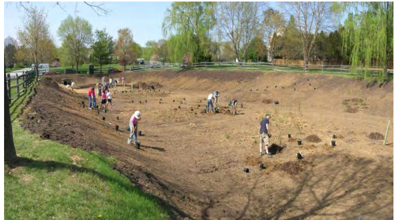
Figure 5.3.13-10. It is important to avoid soil compaction during planting. Retrofit naturalized basins are often good opportunities for volunteer planting efforts if the grading and structural modifications are completed by trained professionals.
