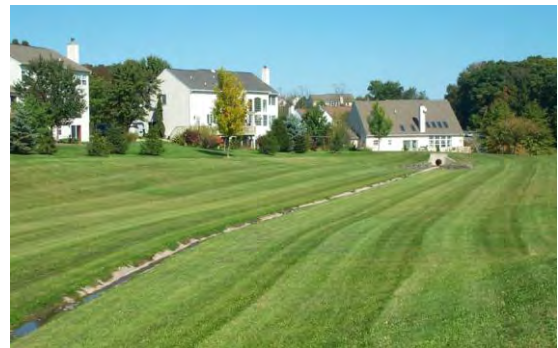
Figure 5.3.13-6. The concrete low-flow channel in this existing basin was removed as part of a retrofit. A meandering, vegetated flow path was created in its place.
