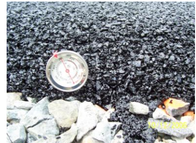
Figure 5.3.1-8. It is important that pervious pavement be placed at the correct temperature as determined by the drain-down test for the asphalt mix.
