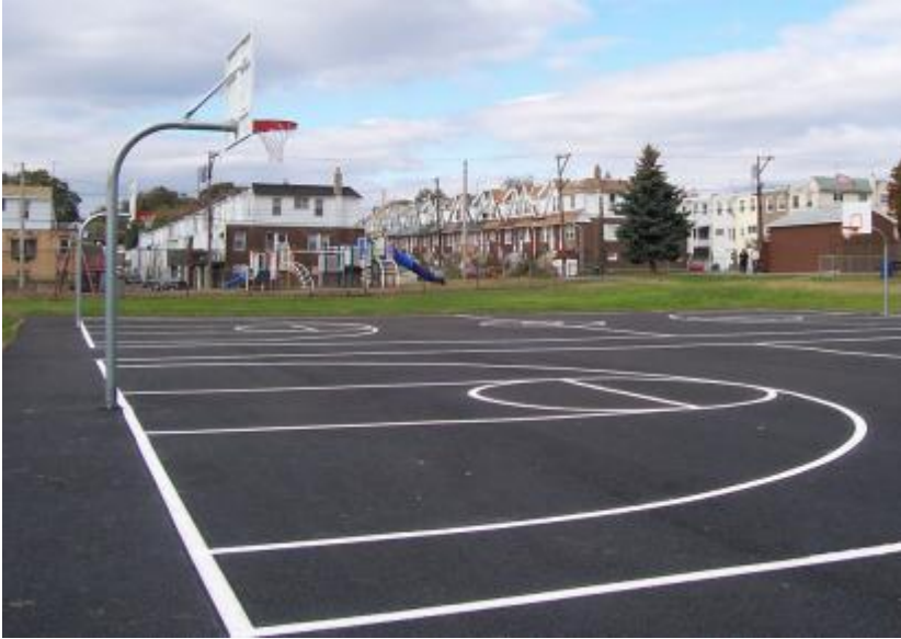
Figure 5.3.1-6. Pervious asphalt basketball court. Pervious asphalt on play surfaces does not form puddles and is quieter when balls bounce.
