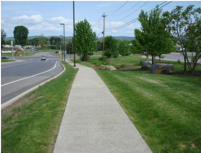
Figure 5.3.1-3. Pervious concrete sidewalk. Constructing sidewalks with pervious concrete reduces impervious area. The sidewalk can also be designed to include a stormwater bed with capacity to receive runoff from adjacent impervious areas (i.e., driveways, roads). This is most applicable where sidewalks are level or mildly sloped (less than 3 percent).
