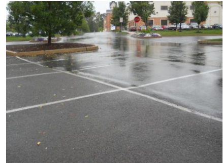
Figure 5.3.1-1. Rainfall drains directly through pervious asphalt pavement (left side of photo) but can be seen as runoff on standard impervious asphalt pavement (right side of photo).
