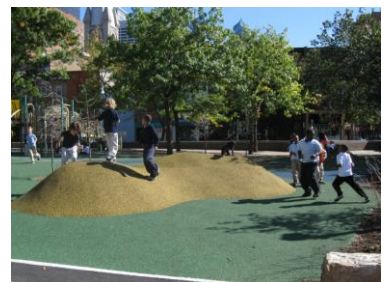
Figure 5.3.1-11. Pervious rubber is an ideal material for a stormwater BMP constructed as part of a playground.
