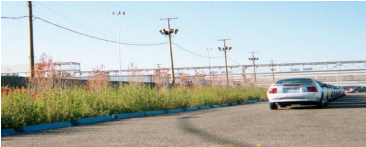
Figure 5.3.5-3. This manufacturing facility includes vegetated swales between parking areas to manage runoff.
