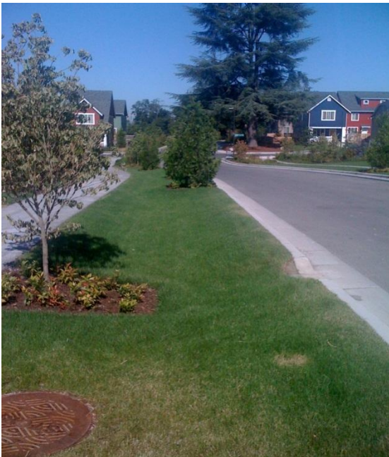
Figure 5.3.5-5. Curb cuts allow street runoff into a vegetated swale in a residential neighborhood.
