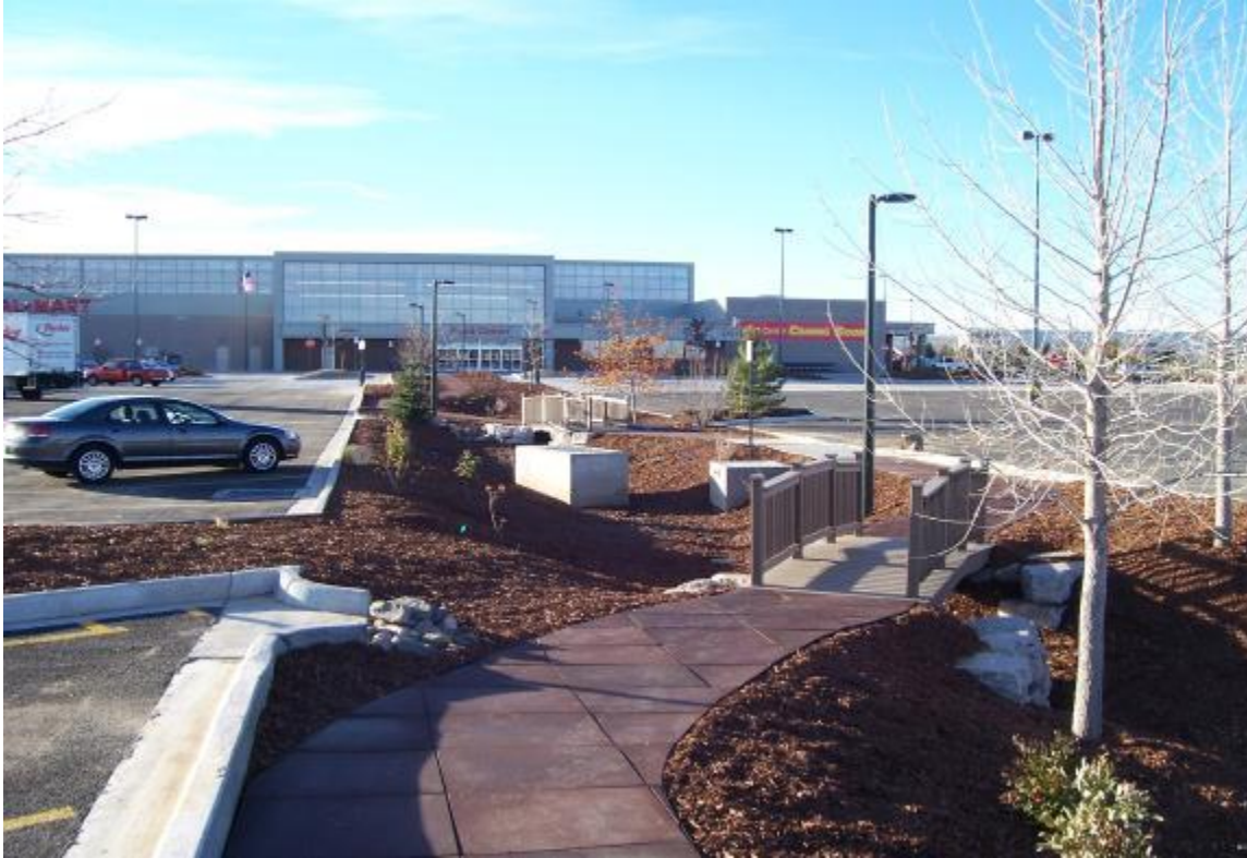
Figure 5.3.5-6. The parking lot vegetated swale at this commercial center is designed for pedestrian crossings.
