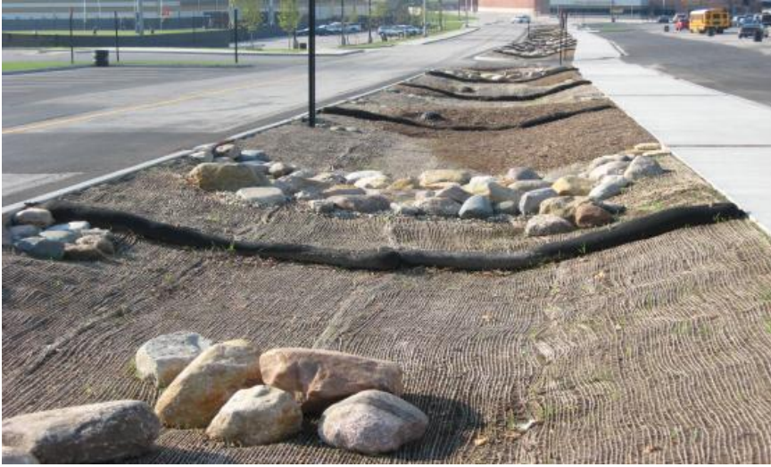
Figure 5.3.5-4. This vegetated swale on a slope includes stone check dams to slow runoff and earthen check dams to retain runoff.
