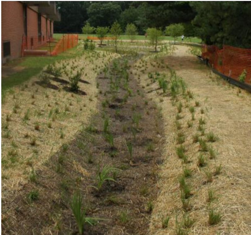
Figure 5.3.5-12. This vegetated swale is stabilized with a temporary turf reinforcement mat until vegetation is established. Careful erosion control is maintained through erosion control materials on the other portions of the site.
