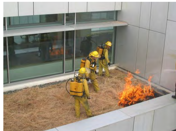
Figure 5.4.2.1-23. Controlled burn on green roof meadow.
