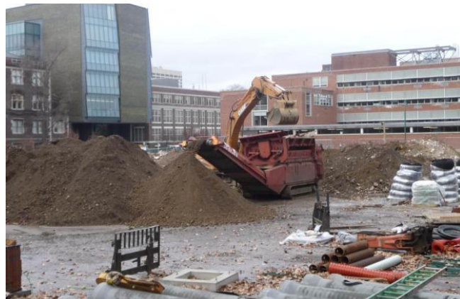
Figure 5.4.3-9. Urban soils being salvaged and mixed onsite.
