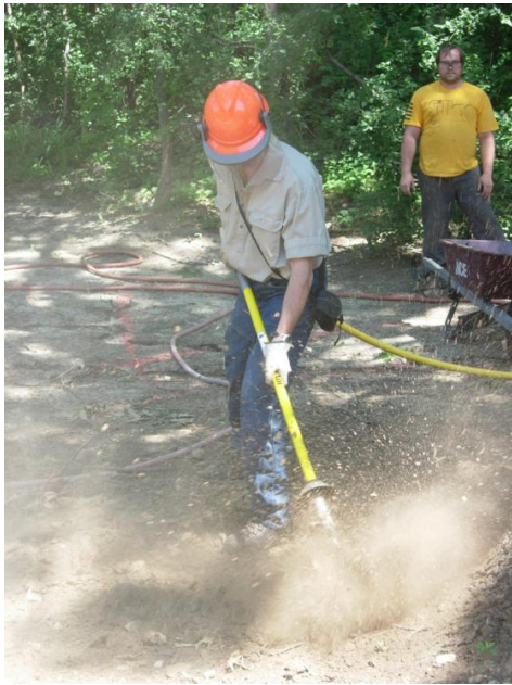
Figure 5.4.3-15. Air spading.
