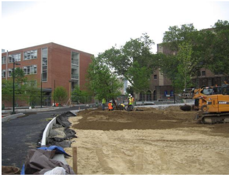
Figure 5.4.3-6. Designed soil layers being installed.
