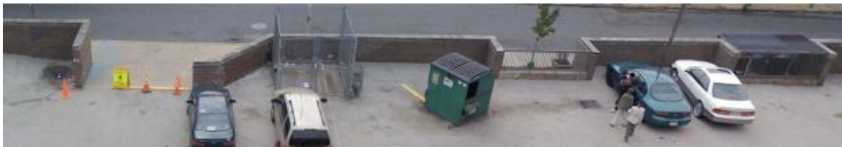
Figure 6-1. Dumpsters and outdoor storage of materials are examples of hot areas that can be addressed through better housekeeping practices.
