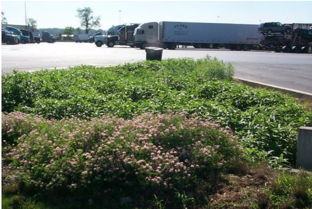
Figure 6-2. Incorporation of a debris and spill containment program at a truck stop “hot area” located atop karst topography with a subsurface infiltration bed. Incorporation of these measures allowed for successful stormwater management, including infiltration on karst.
