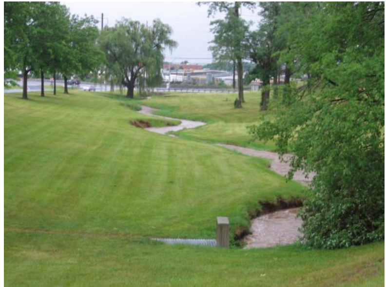
Figure 6-6. A stormwater pipe discharging roadway runoff directly into an urban stream during a rainfall event.
