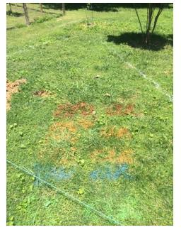
Put in online request for "Call Before You Dig" to clear area to ensure no utilities would be damaged during digging. Free service; took approximately 3 days lead time.
