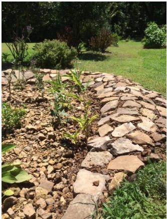
The edges of the garden and berm were then bolstered and strengthened with commercially obtained stones that were placed over the berm and edges of the garden. Gaps between the large stones were filled with sand and pebbles. This took one person approximately 2 hours to place and 1 hour to get pebbles/sand and fill gaps.
