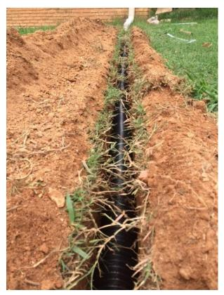
A 4 inch standard pipe pipe was connected to the existing downspout. This took one person approximately 20 minutes with no special tools required. The pipe was then re-buried approximately 4 inches deep. We used a shovel and found a standard push broom to be very helpful to "sweep" the dirt back to the trench. This took 1 person approximately 1 hour to re-bury 55 feet of pipe.
