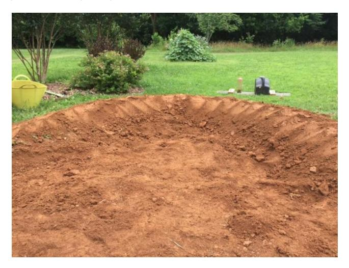
\*At this step, the RainSmart representative was contacted for the subgrade inspection. As the measurements created matched the submitted design, this rain garden passed inspection!
