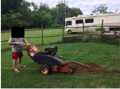
Due to the distance of the rain garden from the downspout, we rented a commercial trencher. The trencher dug a uniform trench for placement of pipe. This required being able to tow a trailer with trencher and operating a large piece of equipment.
