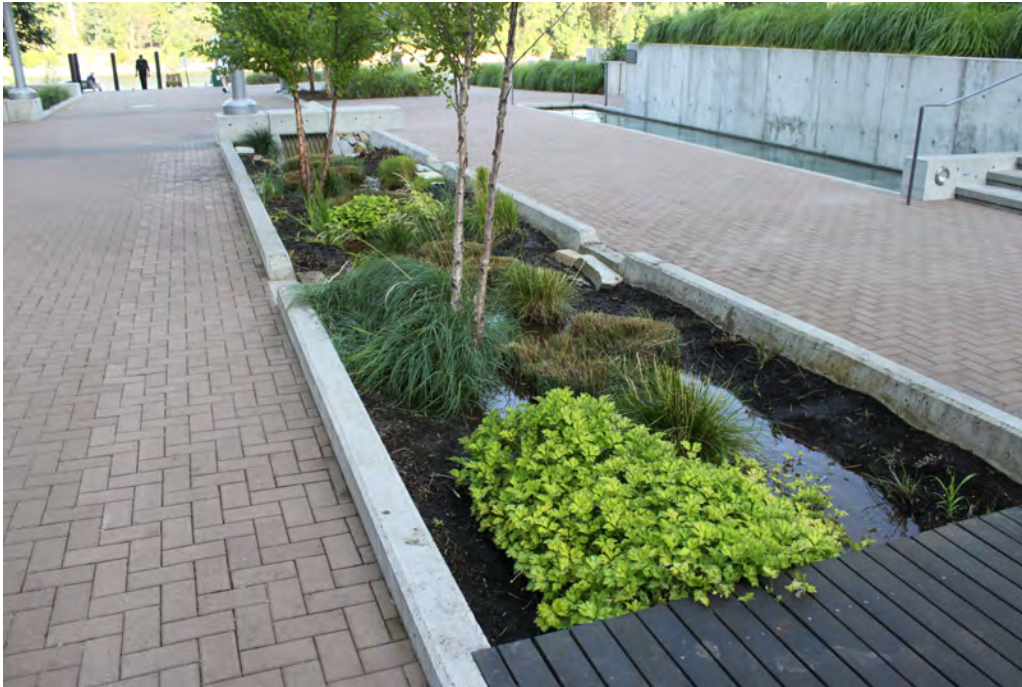
Example of a Stormwater Spine
