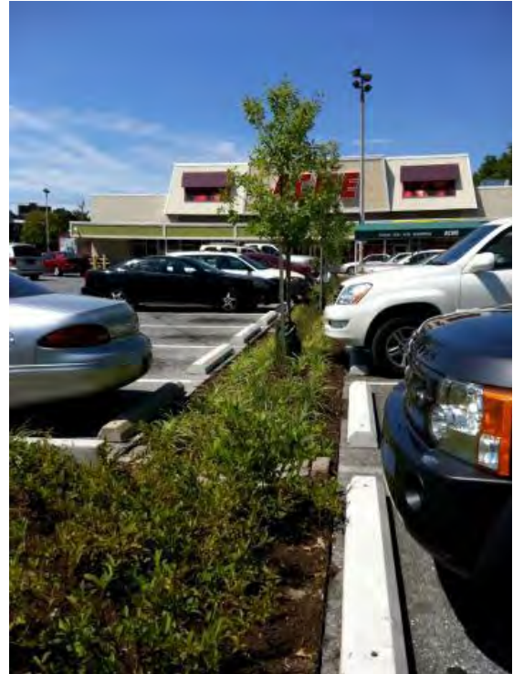
Figure 5.3.4-7. Bioretention in a supermarket parking lot takes advantage of typically underutilized space between parked vehicles.
