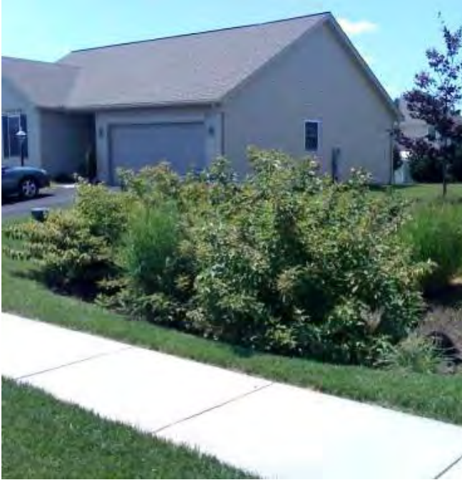
Figure 5.3.4-3. Residential bioretention that manages runoff from a single home. Roof leaders are directly connected to the bed.
