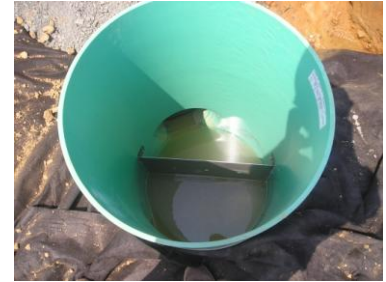
Figure 5.3.1-18. Structures can be purchased with weirs at the desired elevations that allow the small storm volume to be retained while larger flows can safely be conveyed (also see Figure 5.3.1-17).
