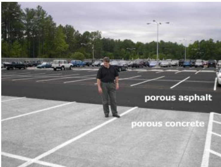
Figure 5.3.1-5. Pervious asphalt and pervious concrete parking lot. The University of North Carolina Chapel Hill park and ride lots include both pervious concrete and pervious asphalt.
