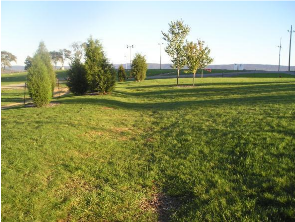
Figure 5.3.3-4. The subgrade storm sewers beneath the lawn at this university campus include infiltration trenches “on-line” as part of the storm sewer system. This is appropriate where the grade is relatively level and the storm sewer is constructed along the contour, as shown here.
