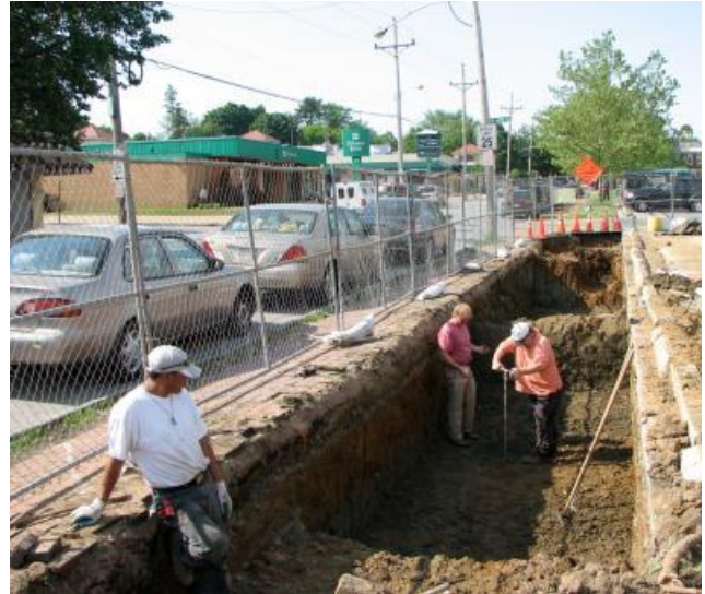
Figure 5.3.3-13. The bottom of an infiltration trench is level and uncompacted. The design engineer should observe conditions before the trench material is placed.
