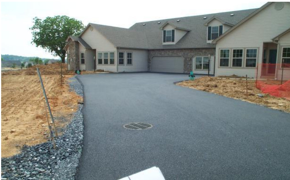
Figures 5.3.2-3a and b. Infiltration beds were incorporated into standard asphalt driveways in this suburban residential development. Standard asphalt was chosen for ease of maintenance and to prevent homeowners from inadvertently “seal coating” porous pavement. Roof leaders convey runoff directly into beds. The sumped catch basin serves to connect the bed to the storm sewer and may also collect driveway and surface runoff. The roof leaders from the house include cleanouts.
