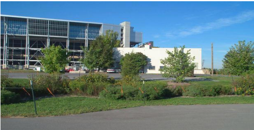
Figure 5.3.2-5. This landscaped area is underlain by an infiltration bed. The bed receives runoff from the upslope impervious areas.
