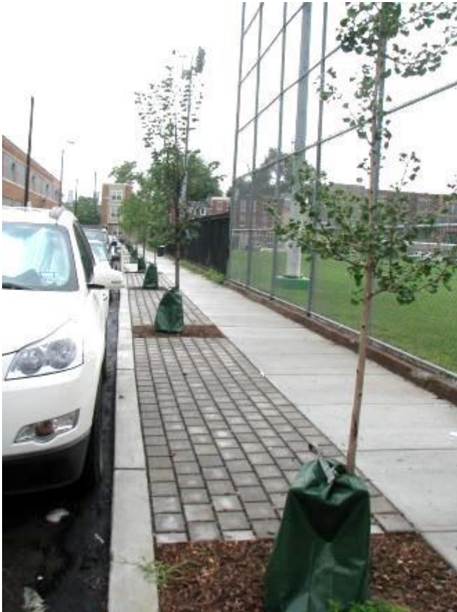
Figure 5.3.3-12. Between the trees in this stormwater tree trench, the soil is extended beneath the porous pavers to provide additional soil volume for the trees.
