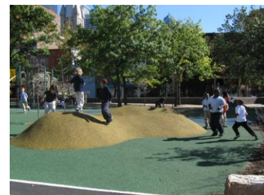
Figure 5.3.1-11. Pervious rubber is an ideal material for a stormwater BMP constructed as part of a playground.
