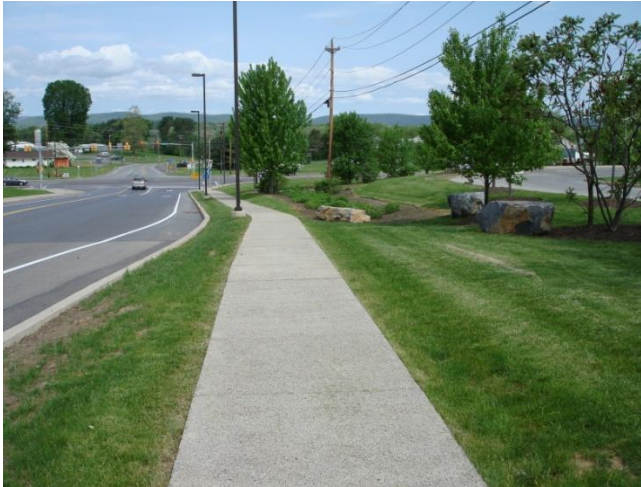
Figure 5.3.1-3. Pervious concrete sidewalk. Constructing sidewalks with pervious concrete reduces impervious area. The sidewalk can also be designed to include a stormwater bed with capacity to receive runoff from adjacent impervious areas (i.e., driveways, roads). This is most applicable where sidewalks are level or mildly sloped (less than 3 percent).
