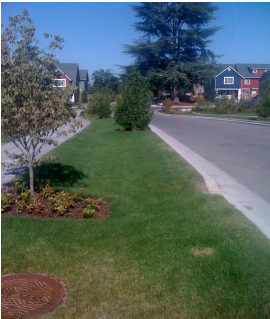
Figure 5.3.5-5. Curb cuts allow street runoff into a vegetated swale in a residential neighborhood.
