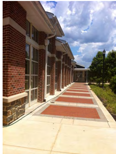
Figure 5.3.4-14. Roof leaders convey runoff below the walkway directly into an adjacent bioretention area. The walk is graded so that runoff sheet flows into the bioretention area. A small filter strip captures any coarse sediment from the walk.
