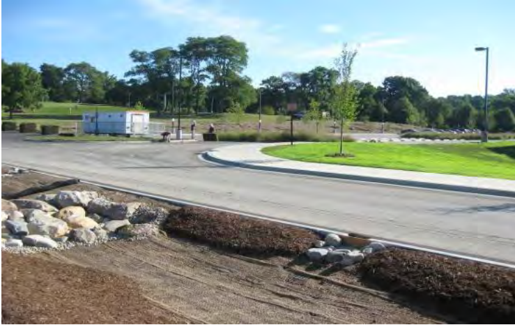
Figure 5.3.4-23. A curb cut is closed to prevent sediment-laden water from entering the bioretention area until site stabilization occurs.
