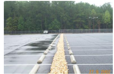
Figure 5.3.1-15. Pervious pavement can be constructed with an unpaved pervious edge treatment. In the event that the pavement is seal coated, clogged, or not functioning, runoff from the pavement can still enter the stormwater bed.
