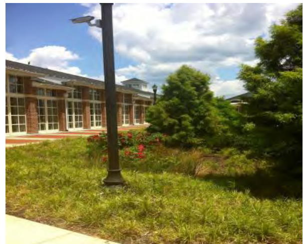
Figures 5.3.4-1a and b. Bioretention area immediately following construction and after three years of establishment.
