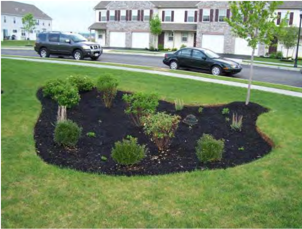
Figure 5.3.4-10. A bioretention area in the public right-of-way avoids homeowner conflicts such as decks, pools, and swing sets and also allows for public access and visibility.
