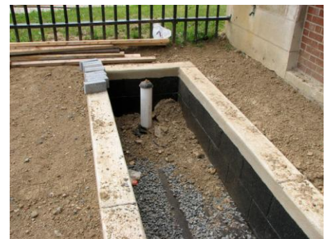
Figure 5.3.11-15. A stormwater planter box that includes a stone bed during construction with geotextile to separate the soil and stone.
