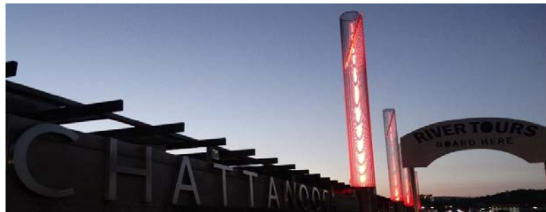
Exhibit 3: Luminous Light Masts (Location: Chattanooga River Pier)
