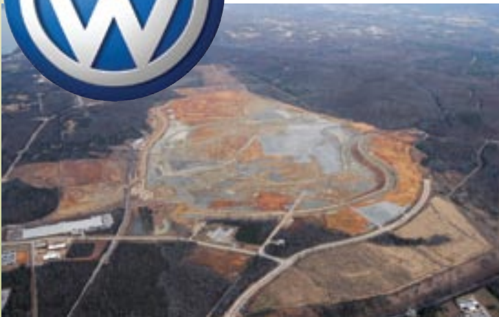
Site preparation for the Volkswagen plant at Enterprise South
