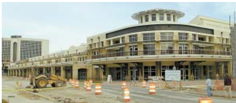
The Chattanooga Trade Center expansion project.
