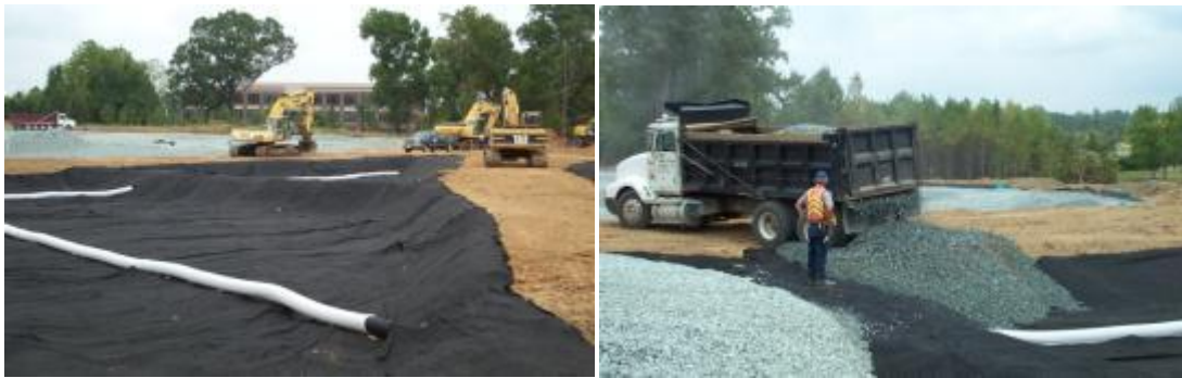
Figures 5.3.1-20a and b. Geotextile and perforated distribution pipes are placed on an uncompacted subgrade, and stone is placed without compacting the bed bottom. Distribution pipes can be designed to extend through berms within the bed.
