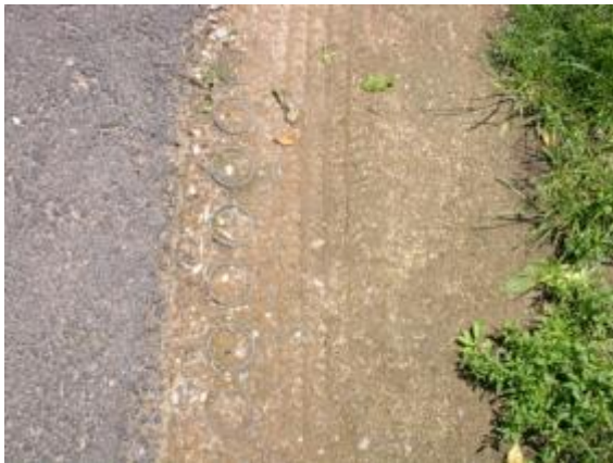
Figure 5.3.1-7-e. Reinforced Turf or Gravel
