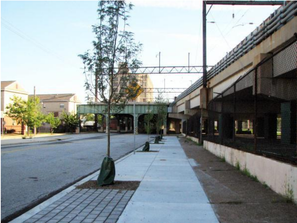
Figure 5.3.3-5. Tree trenches capture street runoff, via curb inlets, and improve urban greening and streetscapes, especially in ultra-urban locations.
