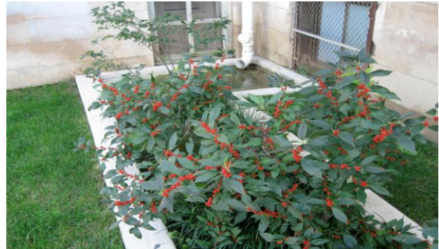
Figure 5.3.11-1. A downspout from an existing building is disconnected to a stormwater planter box.
