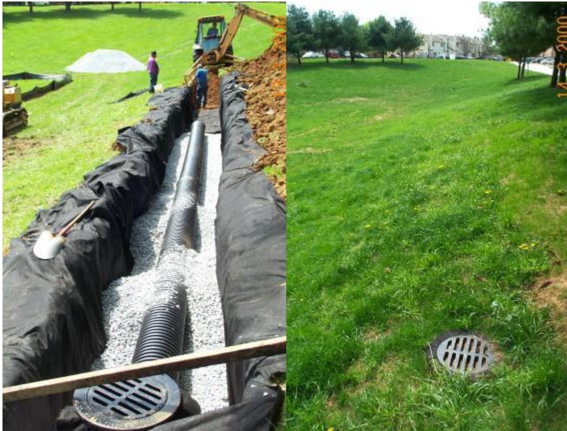
Figures 5.3.3-1a and b. Infiltration trench during installation and afterwards.
