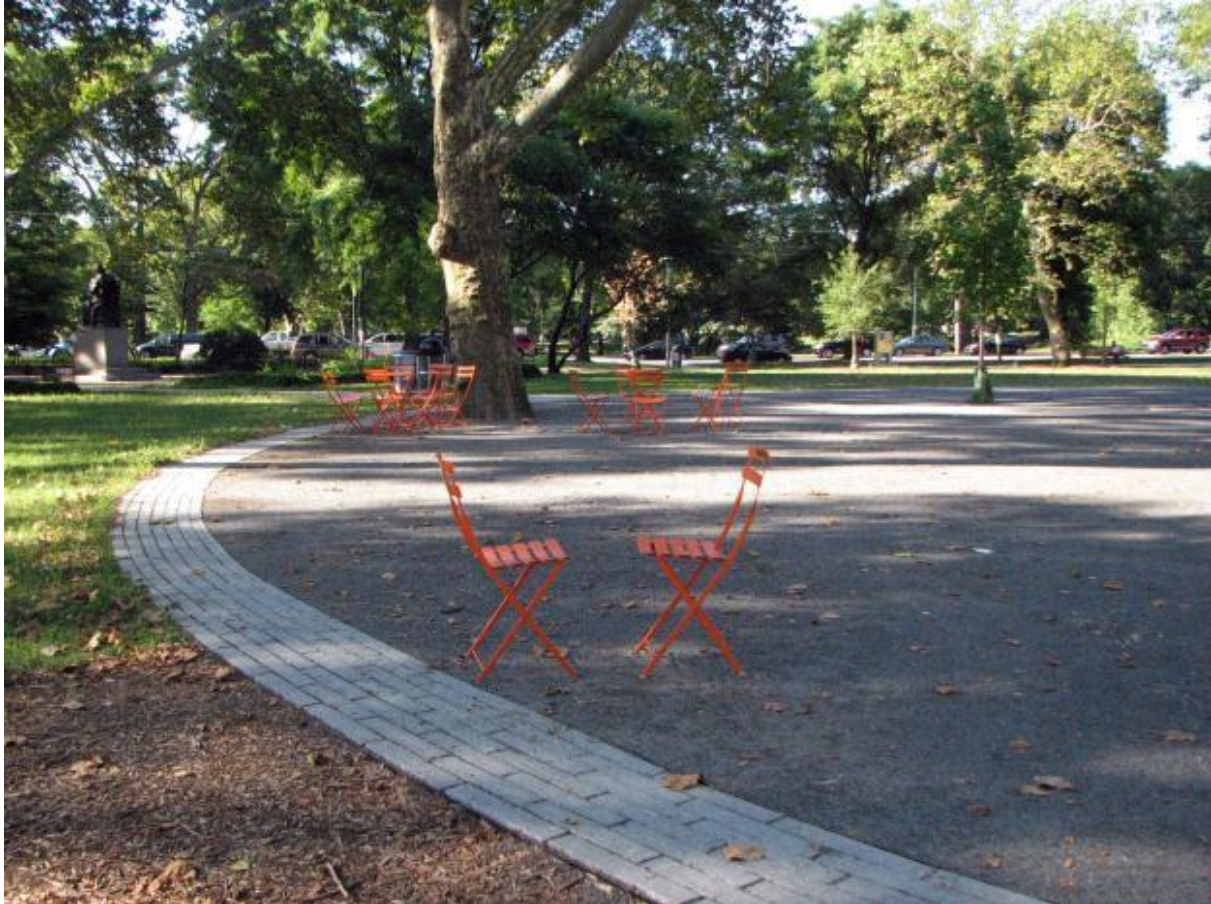
Figure 5.3.2-6. This urban park plaza is built above an infiltration bed that completely underlies the plaza. Runoff is both piped into the bed from adjacent areas and is able to enter the bed through the porous pavers around the perimeter of the plaza.
