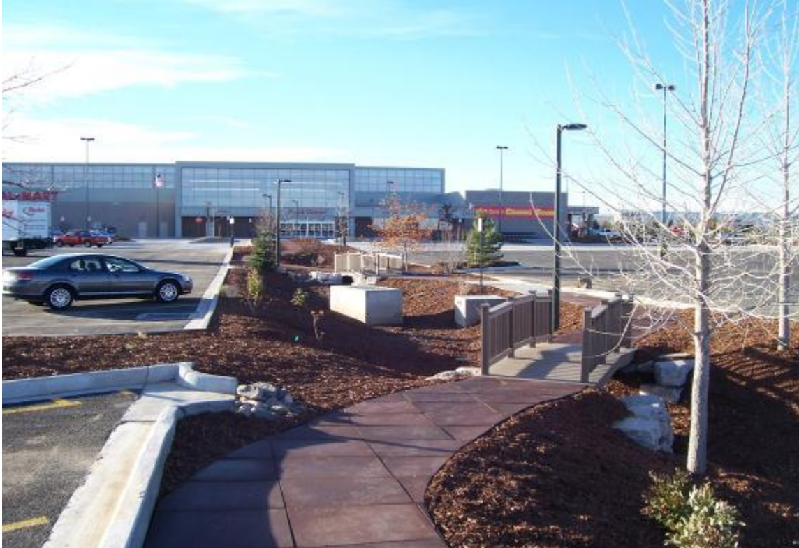
Figure 5.3.5-6. The parking lot vegetated swale at this commercial center is designed for pedestrian crossings.
