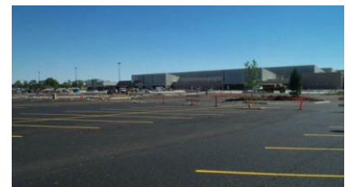
Figure 5.3.1-9. Pervious asphalt at this commercial parking lot includes recycled rubber in the bituminous mix.
