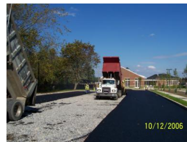
Figure 5.3.1-21: Although the subgrade is uncompacted to allow for infiltration, the stone bed is placed in layers and rolled to provide a suitable subbase for construction vehicles and future traffic loads.
