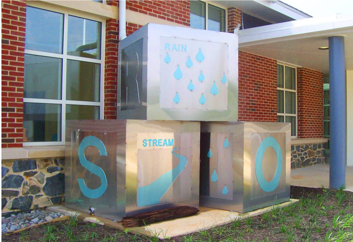
Figure 5.3.9-4. Cisterns can be decorative as well as functional, as is this cistern capturing runoff from a library roof. The cistern, located outside the children’s library, is essentially a rain barrel with a slow-release discharge to the landscape.
