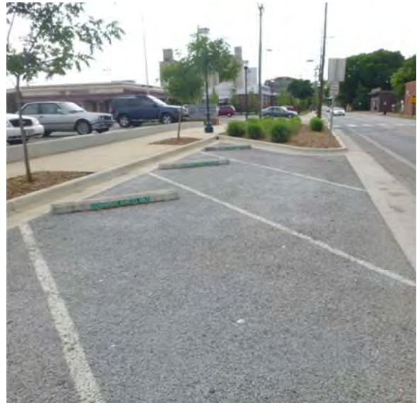
Figure 2-1 11 th Street Police Station Street Parking Pervious Pavement
