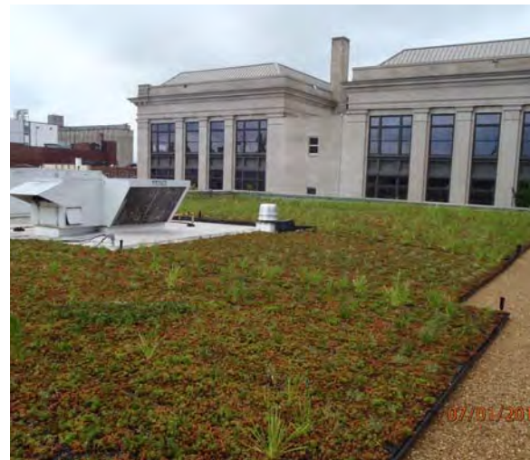
Figure 2-4 City Council Building Green Roof
