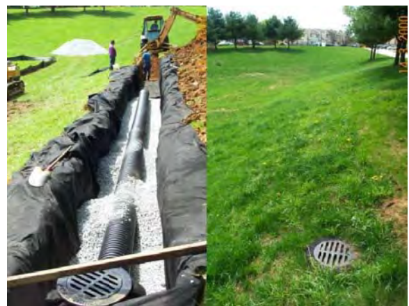
Figure 2-2 Infiltration Trench During and After Installation (RMG Figure 5.3.3-1a and b)
