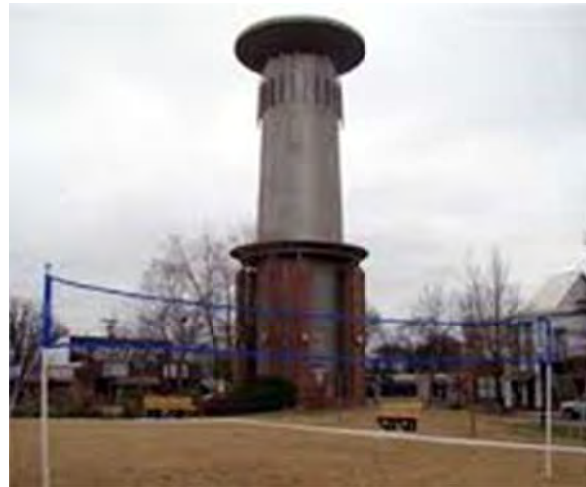
Figure 1-2 17 th Street Water Tower
