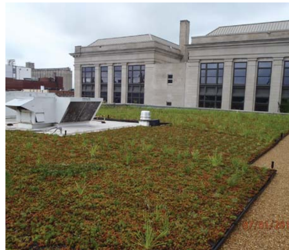
Figure 2-4 City Council Building Green Roof
