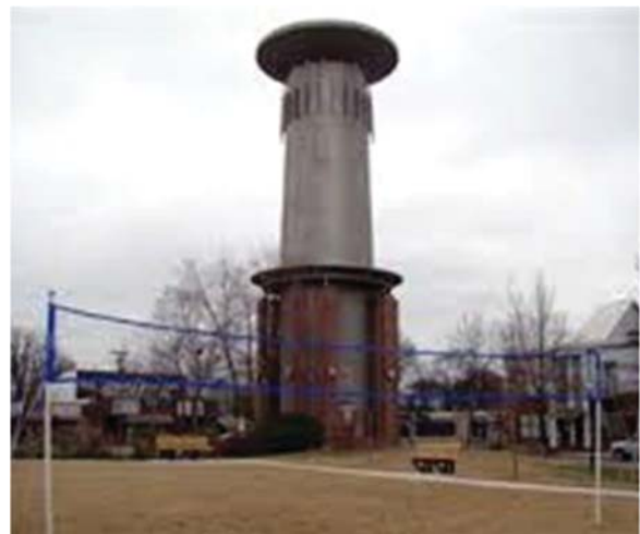
Figure 1-2 17 th Street Water Tower
